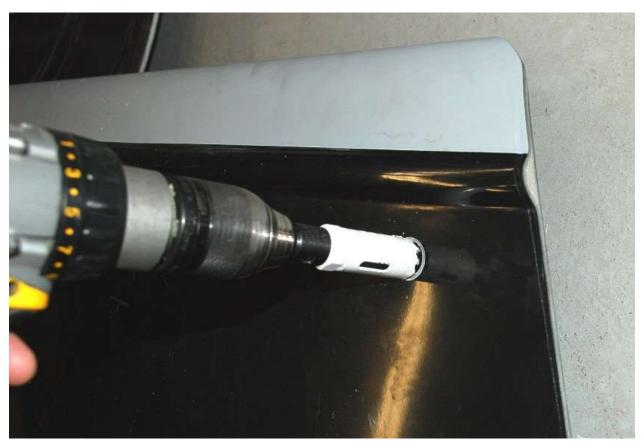
Use  $\overline{a^{7/8}}$ " hole saw on the outer door skin at the point marked.
