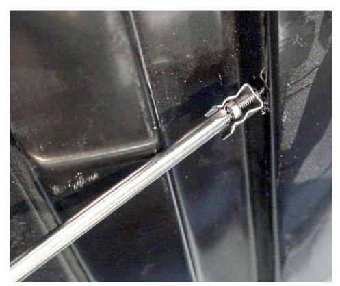
Drill a <sup>3</sup>/<sub>32</sub>" pilot hole and use a self tap mounting screw into fiberglass.
