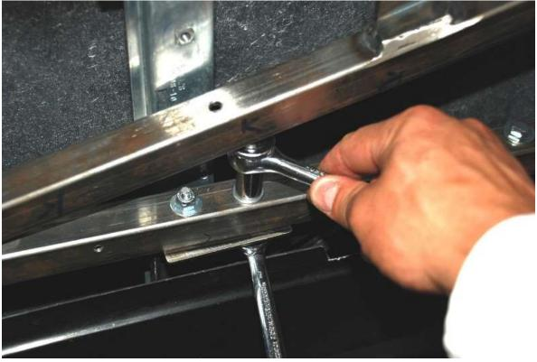
Attach the motor mount bracket to the door frame leaving the bolts slightly loose to allow for adjustment.
