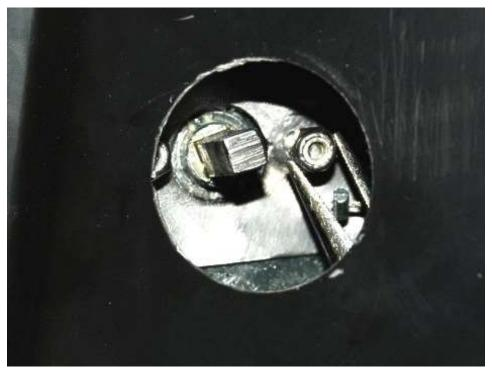
Attach the Handle to the door using the #10-32 x 1" Philip head screws, using a Philips head screwdriver and  $^{3}/_{8}$ " deep socket.
