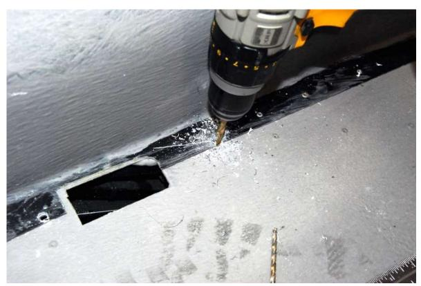
Remove and drill the front hole location with a  $\frac{5}{16}$ " drill bit.
