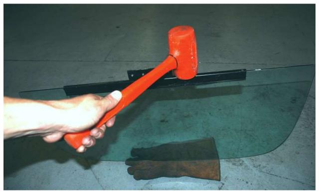
Use a plastic dead blow hammer to push the glass holder onto the glass. Do this evenly on each side of the mount bracket. The last couple of hits will have to be on the mount bracket edge so that it is completely seated.
