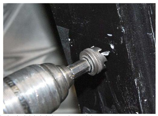
Drill the striker locating hole in the body out using a ¾" hole saw.
