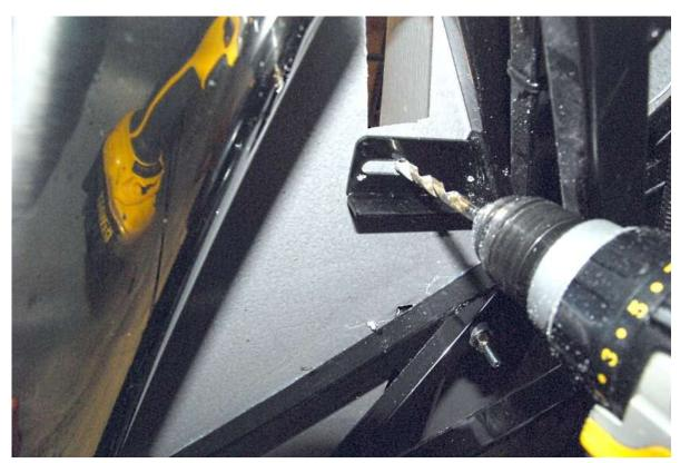
From the under side of the frame, Drill up through the frame e-brake handle mount  $\frac{1}{4}$ " from the inside edge of the slot using a  $\frac{5}{16}$ " drill bit.
