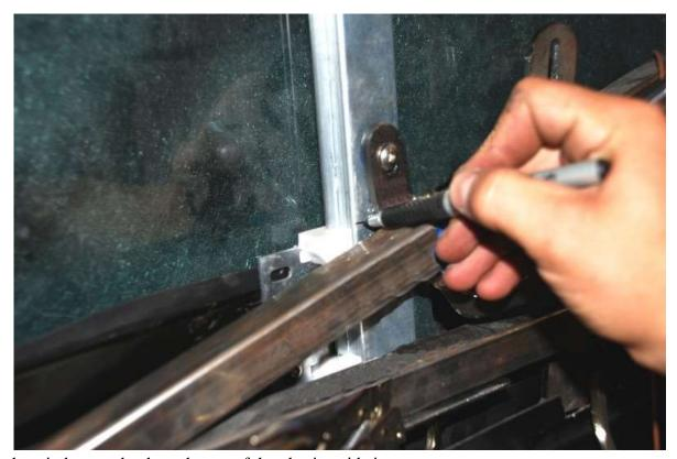
Mark the window track where the top of the plastic guide is.
