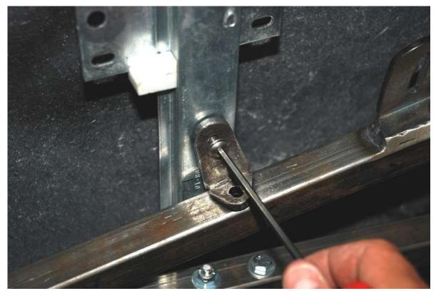
Attach the window track mount to the window track and to the door frame. Leave the bolt a little loose so that the track can pivot on the bolt if needed and so the bottom can move in and out.
