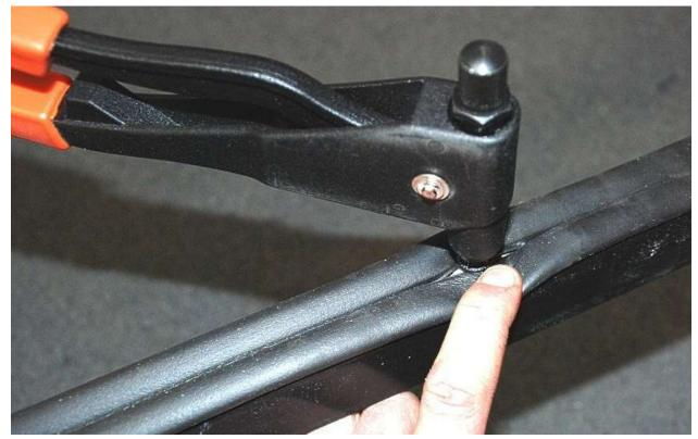
Insert and attach 1/4" rivnuts in the 25/64" holes just drilled.
