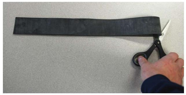
Fold the 36" piece of window channel rubber in half and cut it in half. One piece will be used for each door.
