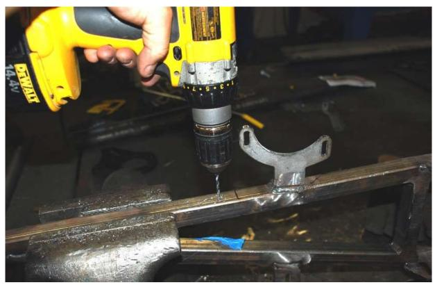
Use a ¼" drill bit to drill through the tube at the hole locations marked.
