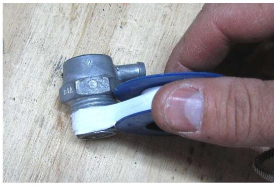
Wrap the vent with Teflon tape
