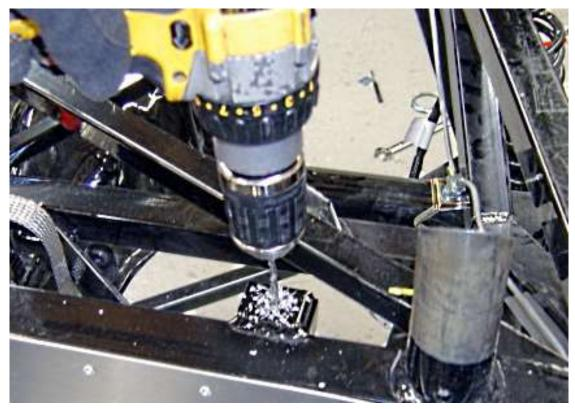
Remove the tank and drill the (4) mount locations on the frame tabs with a 3/8" drill bit.
