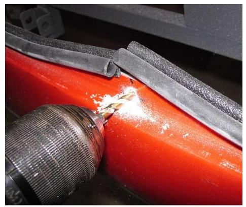
Drill the body location with a <sup>3</sup>/<sub>16</sub>" drill bit.
