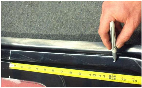
Measure out from the hood center 12" on each side and mark the middle of the hood liner rib for the hood handle location. If the hood sticks up slightly at the corners, change this measurement to 13"
