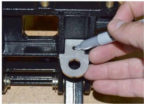
Place the switch mount between the brake pedal mount tabs on the side closest to the brake pedal pivot holes and drill a  $\frac{3}{16}$ " hole through the brake switch mount hole and the pedal box.
