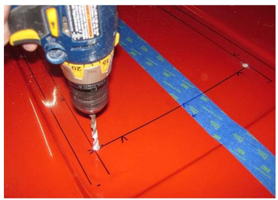
Drill 1/4" holes at the front corners of the area marked
